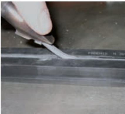
– Installation of Datwyler Black Swell into the composite Tunnel Gasket
