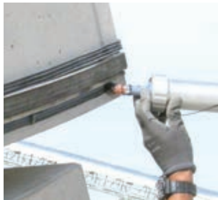
– Installation of the Datwyler Black Swell Gasket Frame with Datwyler FP-75
